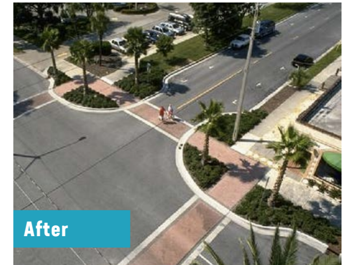
Organised intersections with clearly marked pedestrian crossings, tactile paving and garden beds.
